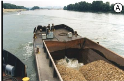
Testing of granulometric river bed improvement with coarse gravel
