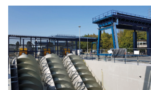
Renewable energy & smart water use at locks
